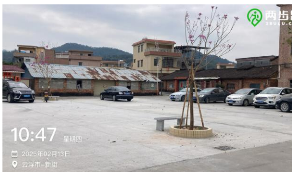
拆除铁棚鸡舍或微修缮
